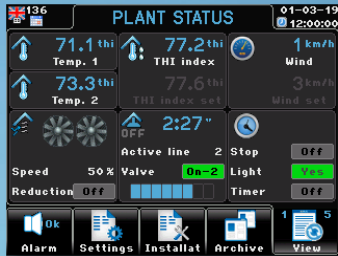
Viewing operating condition
